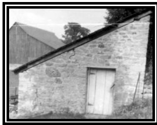
Ice house in back of home. A stream ran through it to keep food cool
