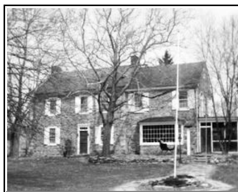
Back of LeVan home/mill
